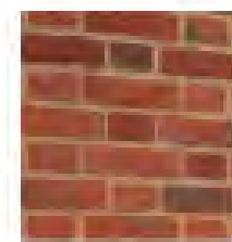
LOWER WALLS BRICK
